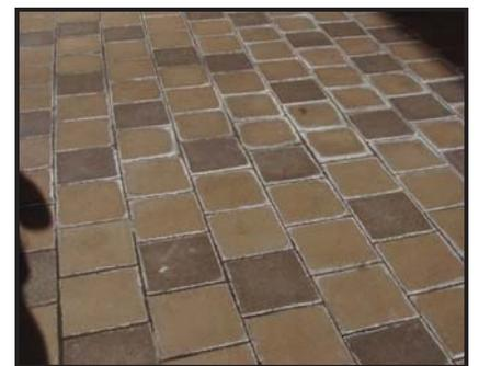
If the masonry element is exposed to large concentrations of moisture such as rain or snow during construction, but prior to hydration, setting and bonding of the mortar and grout, the salts in the materials are more susceptible to being dissolved.
