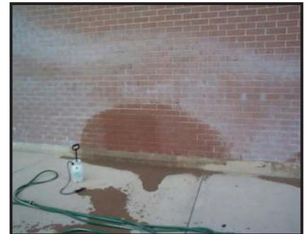
If the salts are not water soluble, attempt to identify the type of salts present. Consult the masonry manufacture for assistance in identifying free salts. Vanadium and Manganese are salts inherent in many buff and brown and black colored brick. These and other salts may require special cleaning agents to remove them.
