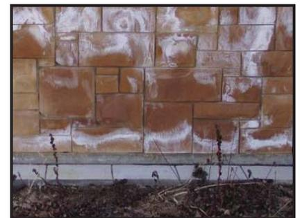
Some “not effloresced” brick have higher absorptions. The higher absorption brick allow more water to enter the masonry which provides more water to
