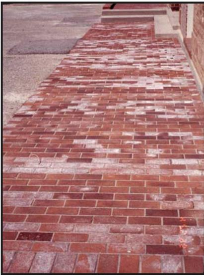
High vapor transmission rate (VTR) water repellents have been known to help in reducing efflorescence by reducing the amount of water that gets into a wall thereby reducing the amount of solution available to dissolve the salt. Water repellents also help in reducing the rate of evaporation which slows down the flow of water in the wall which reduces the transportation of larger particles.
