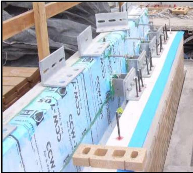
structural brick, the panels could be constructed in place which eliminated added costs in freight, labor and handling. Each wall was built as a panel separated by vertical and horizontal expansion joints. Although built in place, each panel was connected to 4 heavy Galvanized Steel Plate connectors that carry the vertical and lateral wall loads. Connectors are designed similar to precast panel connectors with allowances for in-plane vertical and lateral expansion, contraction and deflection.
