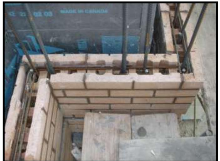
sufficient cell space to allow for reinforcing and grout. The brick coring is larger and configured so that the cells align and can be reinforced when placed in the wall bond pattern. Reinforcement increases the structural capacity of the brick wall. This allows the spacing of wall ties to be increased to distances between floors and columns. Conventional veneer ties are thus eliminated and replaced by more substantial connectors.
